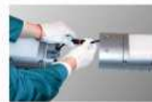
Connect the waterproof plugs
